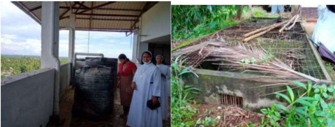
Figure 23 RAIN WATER TANK FOR TOILT FLESH & WELL IN BACK SIDE OF AUDITORIUM
